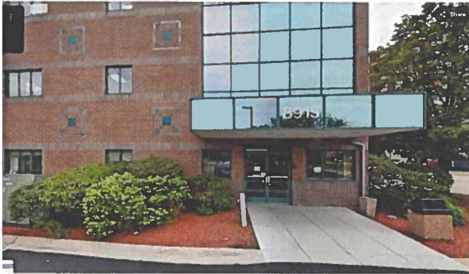
Street view of property 8915 West Golf Rd, Niles, IL 60714
