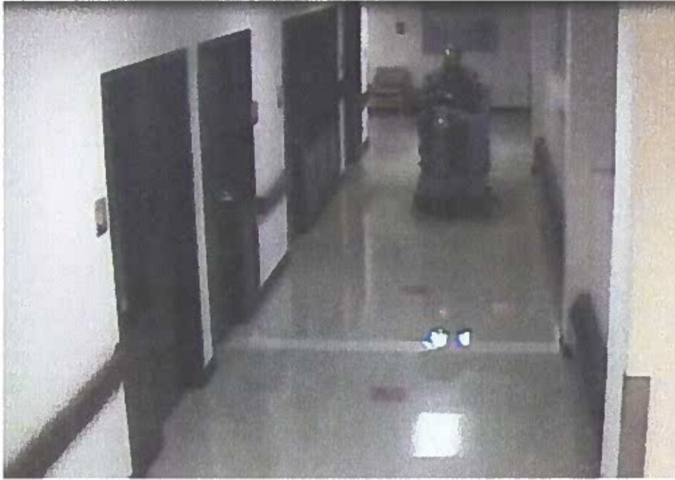
Figure 3: Image shows inside Javon Bea Hospital – Rockton 15 minutes later as water starts filling the basement of the hospital.
