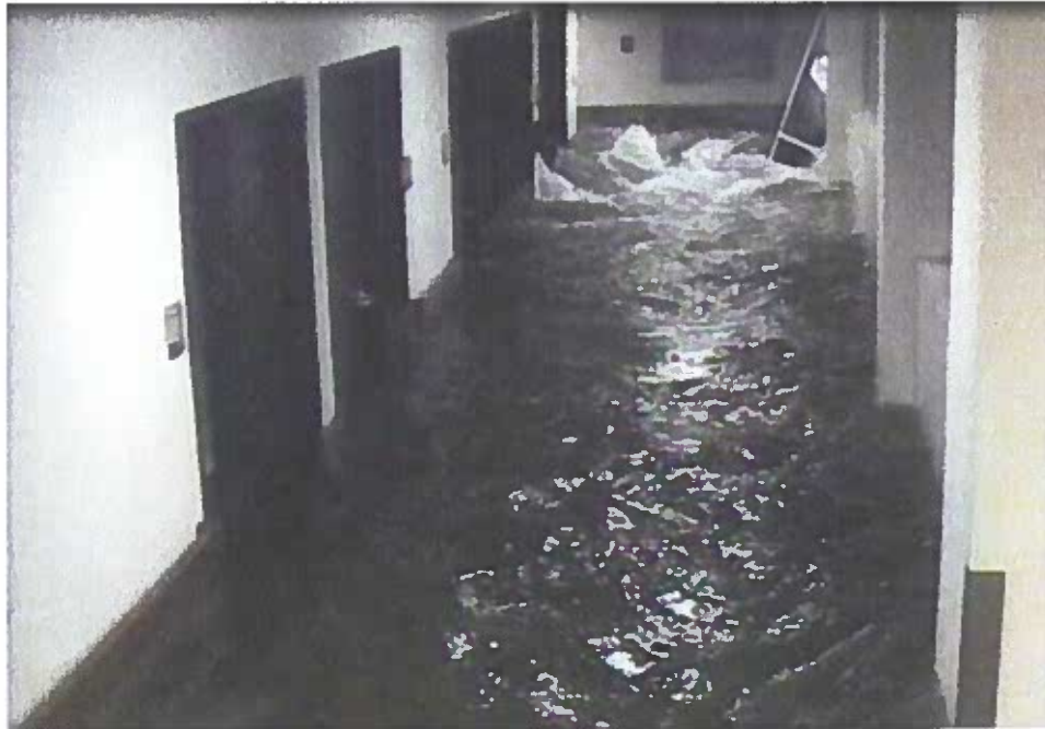
Figure 5: Image shows inside Javon Bea Hospital – Rockton 20 minutes later with water levels risen to nearly two feet in the hallway of the basement.
