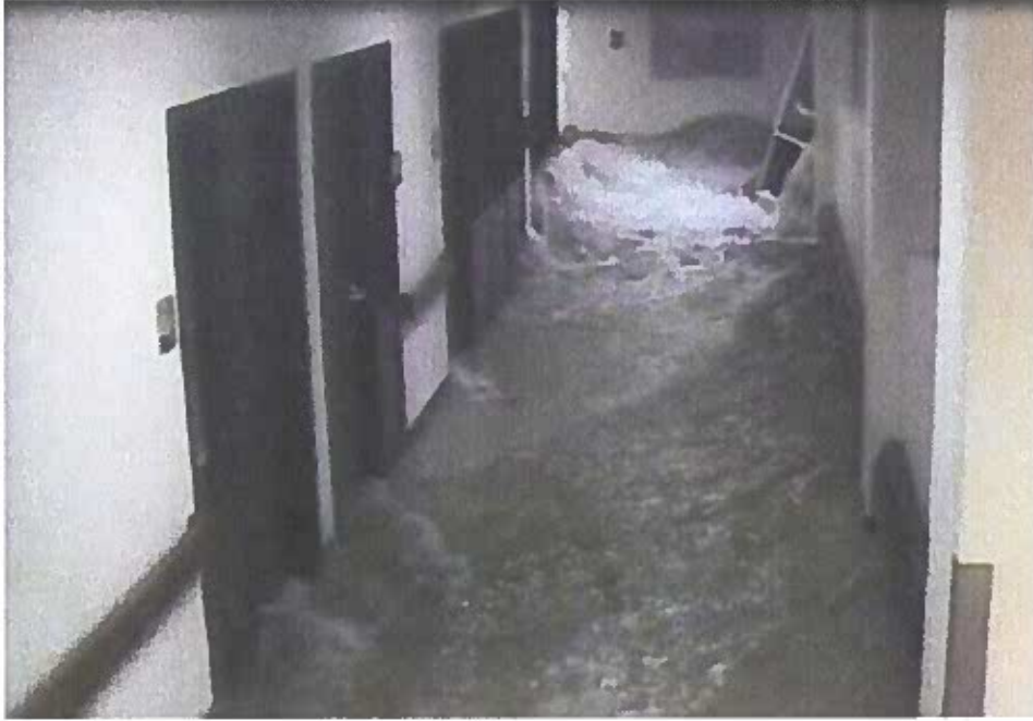
Figure 4: Image shows inside Javon Bea Hospital – Rockton 5 minutes later with water rushing through the basement after the external courtyard was fully engulfed in water which led to windows breaking and massive amounts of water entering the building.
