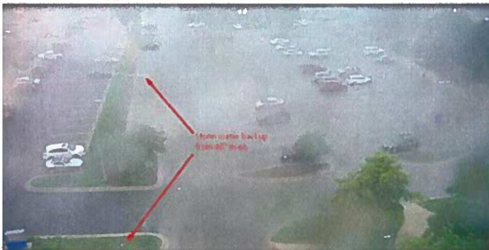
Figure 1: Image of Rockton Campus Parking lot with arrows indicating locations where the storm water backup happened from the 48" main entrance.
