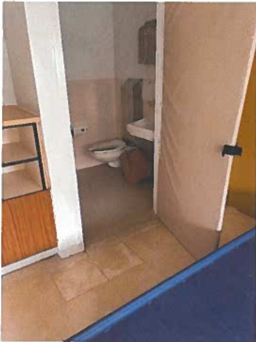
Discoloration of floor tiles from lifting from water
