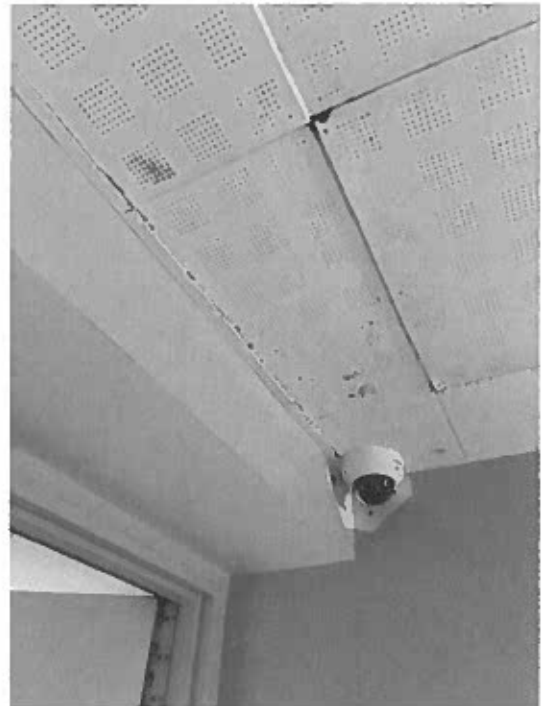
Condensation down the walls from radiant heat above
