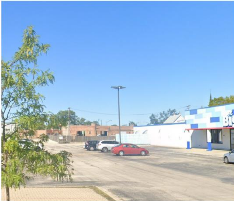
Rear View of Building at 7403 Milwaukee Avenue, Niles, Illinois, 60714
