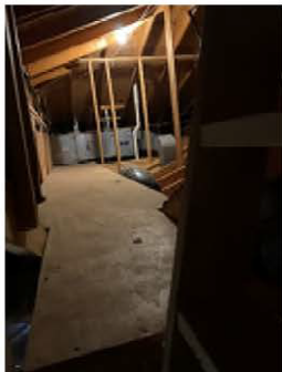
Attic – catwalk system with Air Handler unit imbedded in truss areas.
