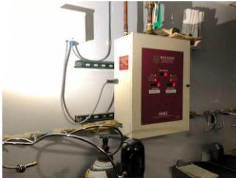
Two banks of Nitrous Oxide in medical gas room.
