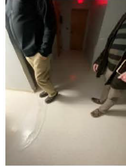
Floor damage present in restricted corridor.
