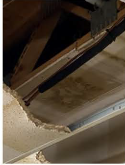
Basement – visible water damage and holes in required floor ceiling assembly rating between basement and first floor.
