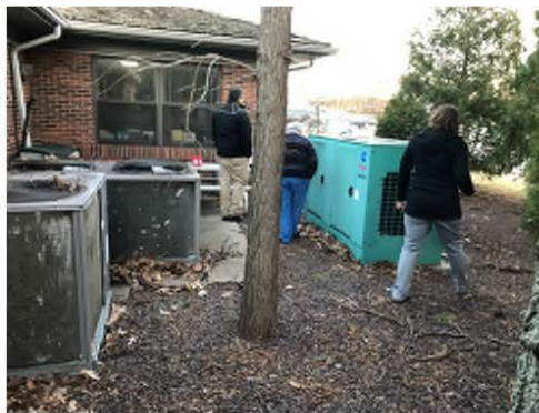
Condensing units and one of two emergency generators.
