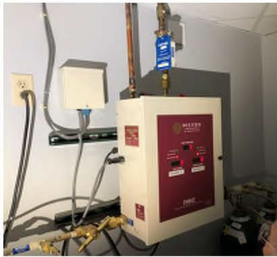
Two banks of Nitrous Oxide in medical gas room.
