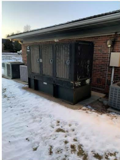
125KW Diesel Generator
