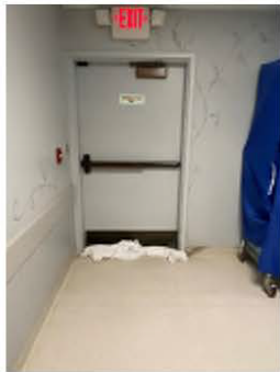
Exterior door with towels underneath (likely water and / or air infiltration issues).
