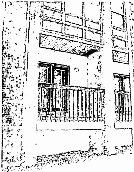
71. EIFS at balconies at apartment building needs to be cleaned and elastomeric coating applied
