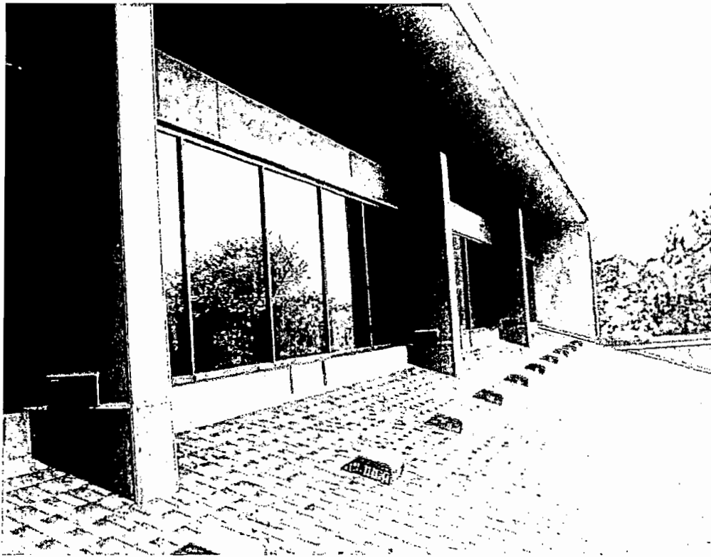
48. Storefront windows provide natural light in atrium of apartment building
