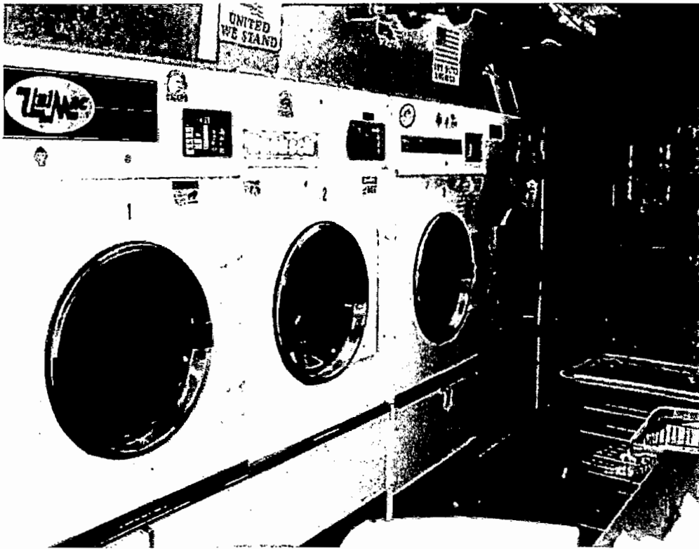
131. Five commercial dryers are located in the basement laundry
