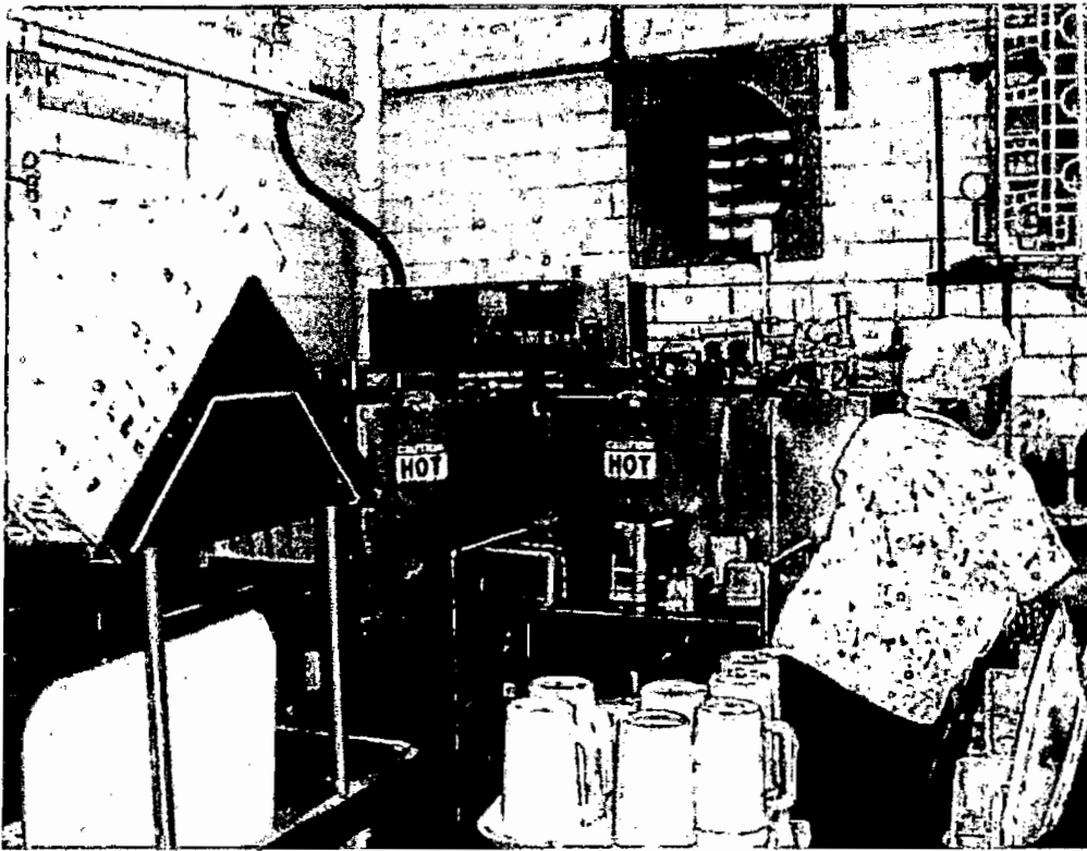
110. Thru-wall fan evacuates water vapor from Shelter kitchen dish room
