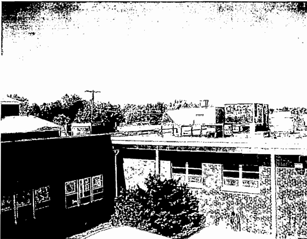
147. From left to right, packaged heating and cooling unit for Shelter Care dining room, makeup air unit (with electric heat) for Shelter kitchen, and packaged HVAC unit for kitchen
