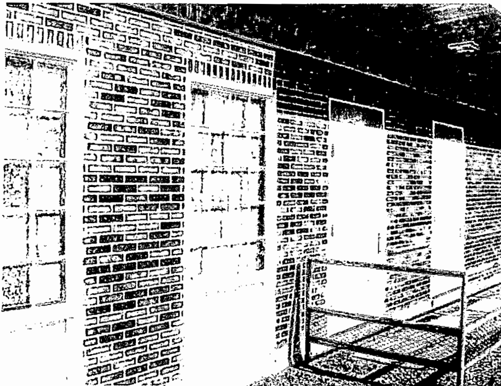
130. Frames at stained glass windows and emergency exit doors at chapel need to be cleaned and painted
