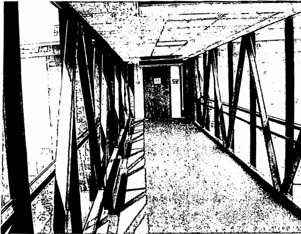
10. Two split DX systems and four heat strips provide heating and cooling for pedestrian bridge
