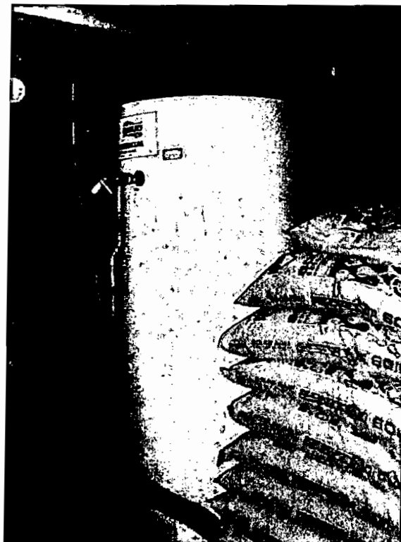
138. Domestic hot water storage tank in basement of Shelter Care
