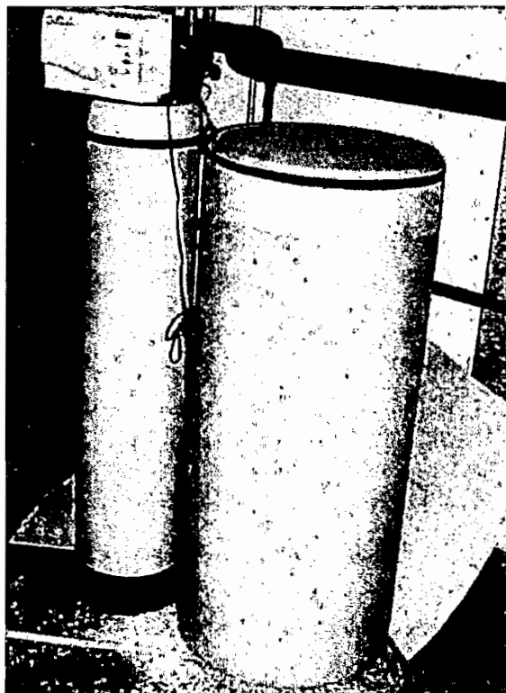
37. Water softener is provided for domestic water treatment in the ILU apartment building
