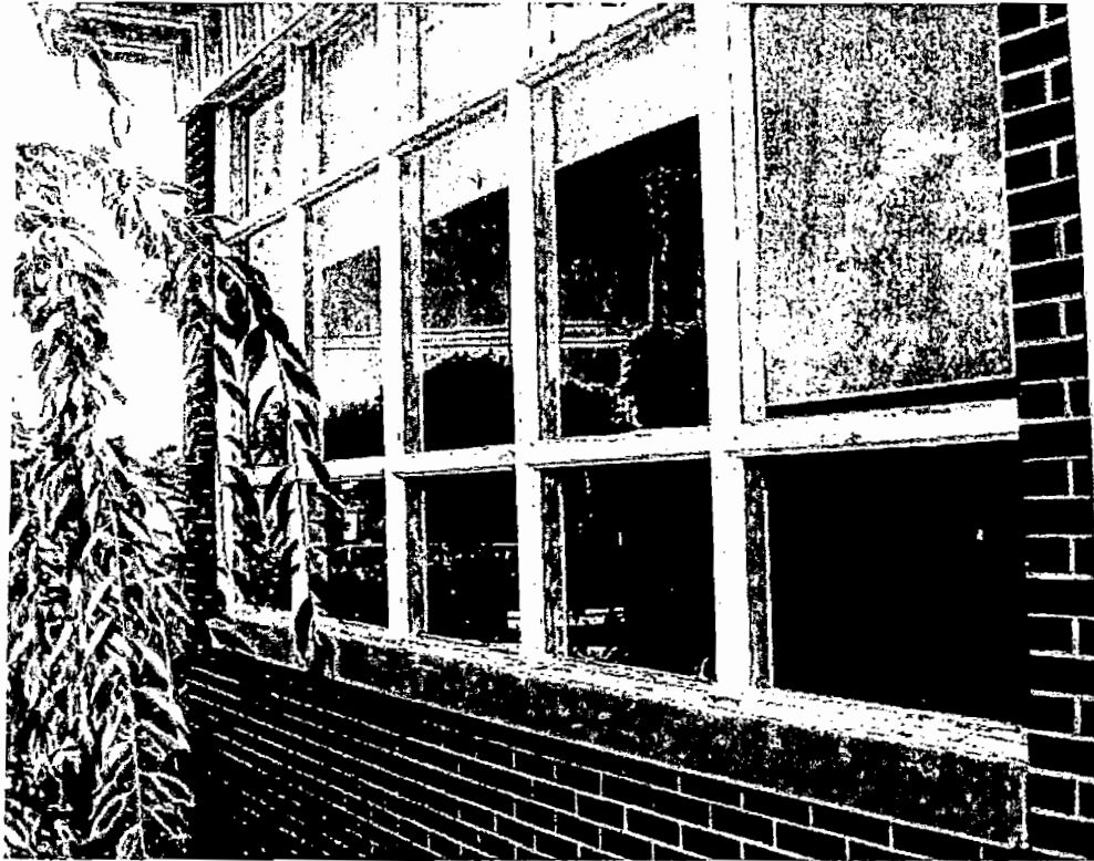
100. Fixed sash windows on south elevation of Kohl Wing need to be replaced
