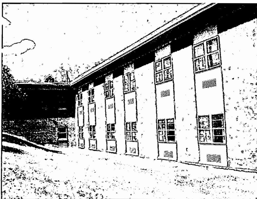
124. West elevation of Roediger
