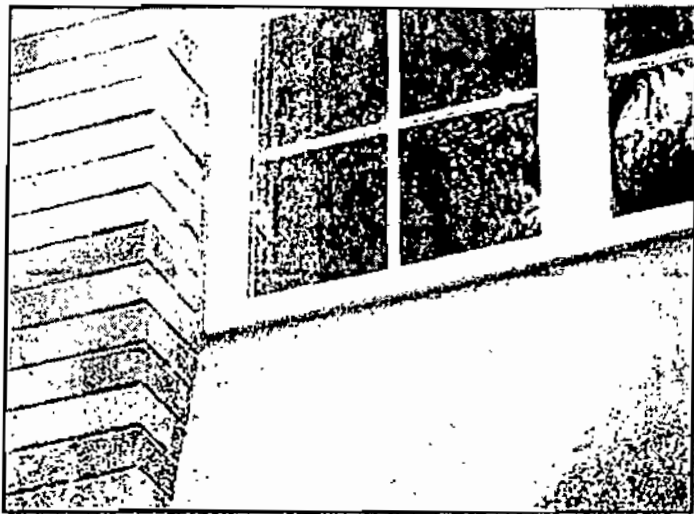
Sealant at Building B. Olson - note deterioration
